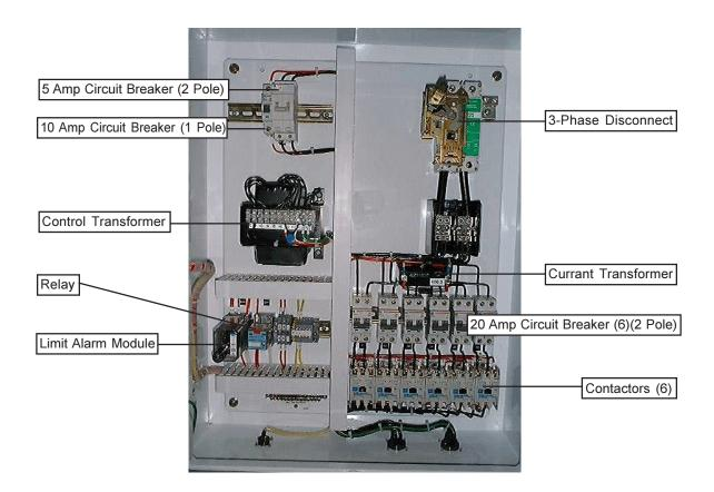
The 603712.B heater control unit controls up to (24KW) 120 amps, divided into six (6), (4KW) circuits, at 230 volts, single (1) phase.
